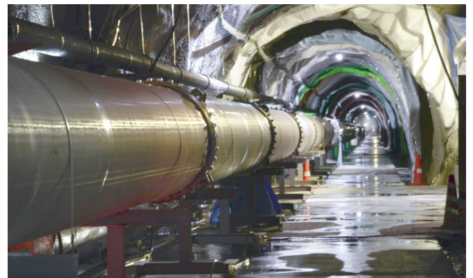
Fig. 1: One of the 3 km arm ducts of KAGRA.
